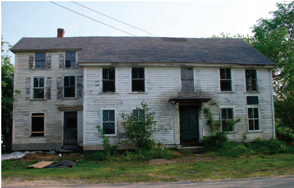
Figure 2. The Barrett Farm house in 2007. View is to the north.
