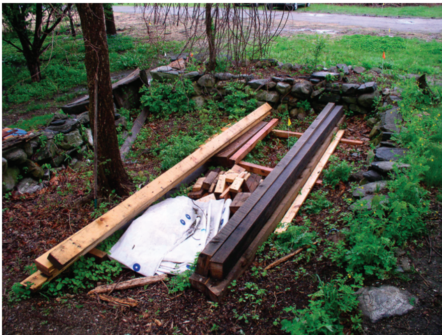
Figure 5. The remaining exposed east ell foundations.
