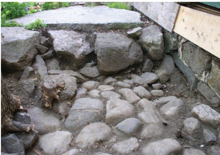
Figure 28. East ell cobbles continue under the surrounding fieldstone foundation. View is to the south.
